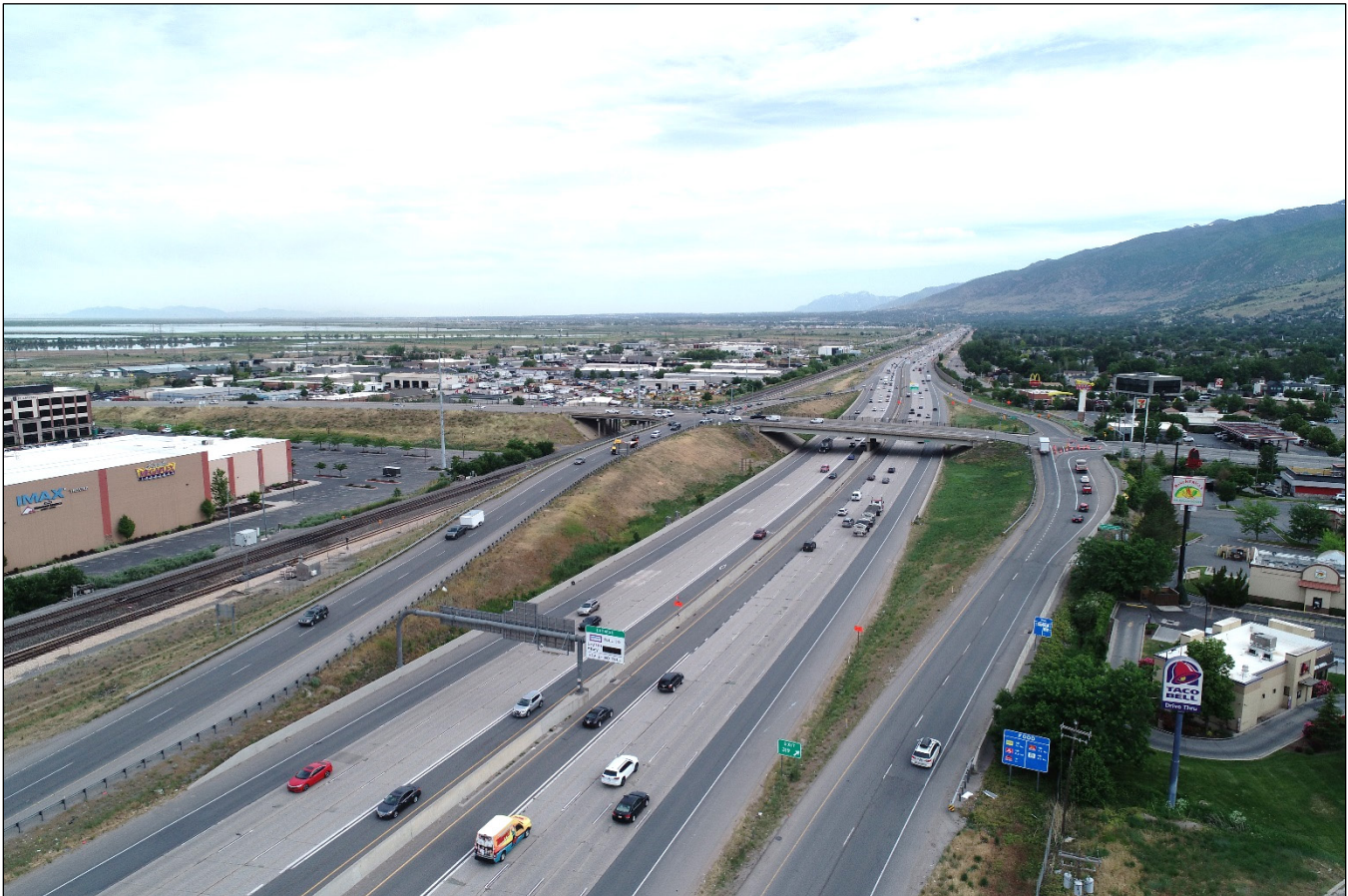
Figure 3.15-10. Key View 3 Looking North over the Parrish Lane and I-15 Interchange
