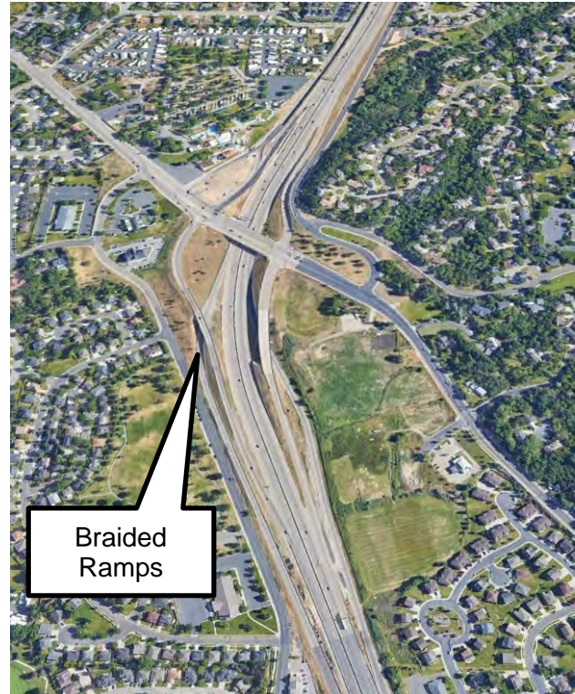
Figure 3.15-15. Braided Ramp Example on U.S. 89
