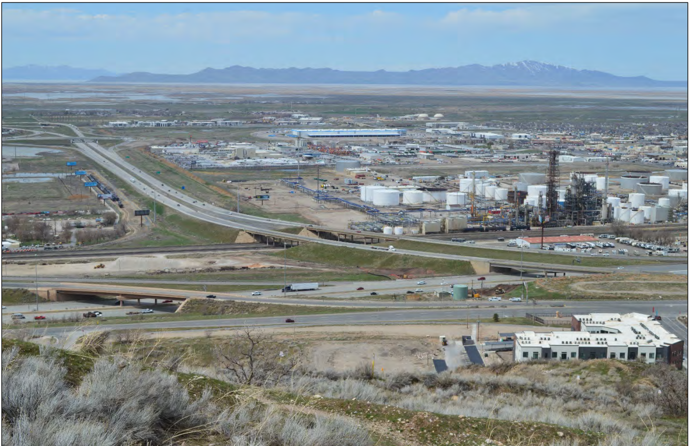
Figure 3.15-12. Key View 5 Looking West across U.S. 89, I-15 and I-215 in North Salt Lake
