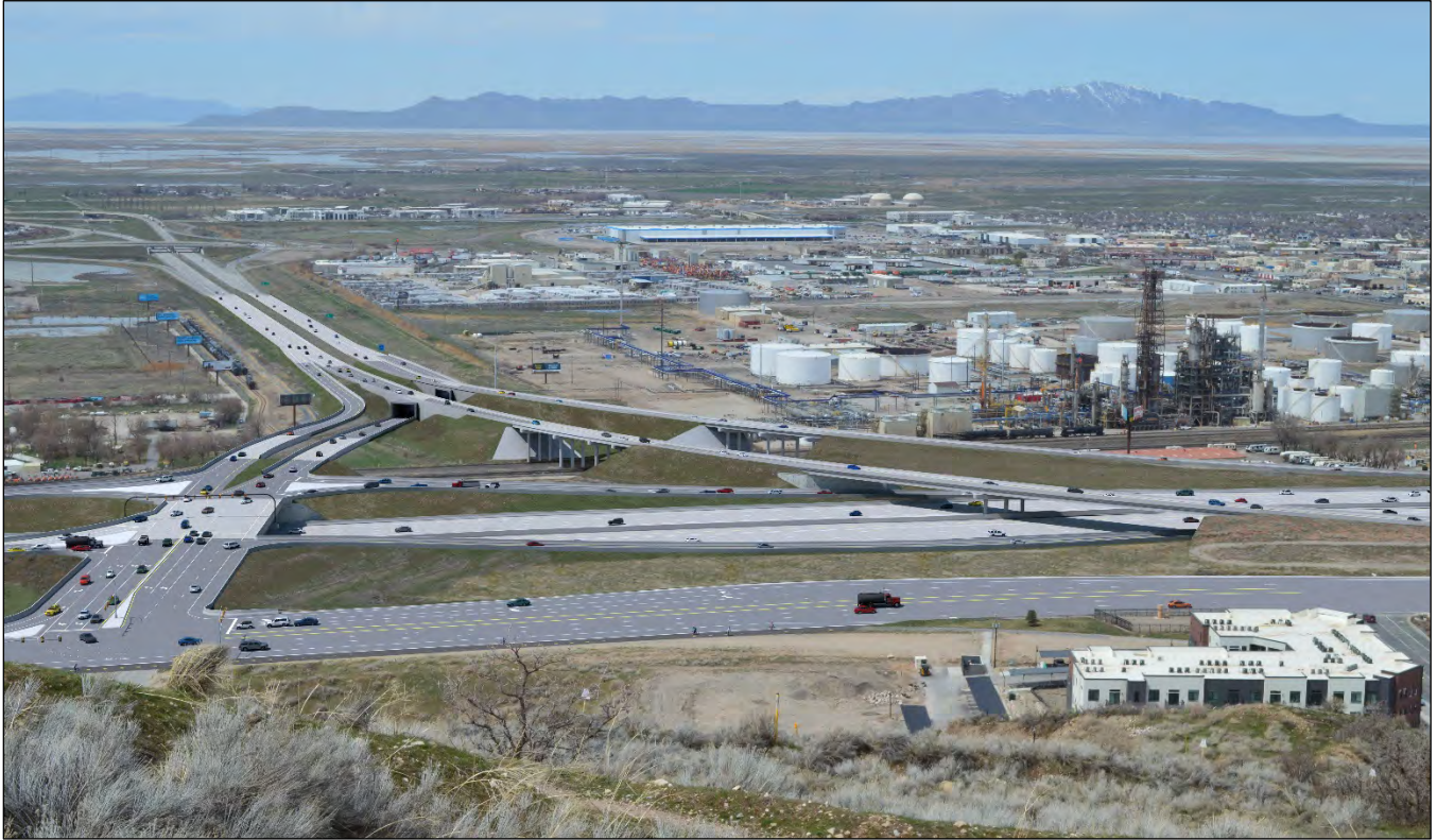
Figure 3.15-18. Key View 5 with Simulation of the Action Alternative at the New U.S. 89, I-215, and I-15 Interchange
